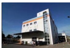
Commissioning of the PCE plant in Bottrop
