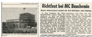
Construction of production and administration facilities in Bottrop
